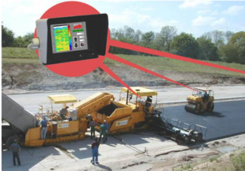
**Figure 4. Continuous Asphalt Compaction on BAB A20.**
